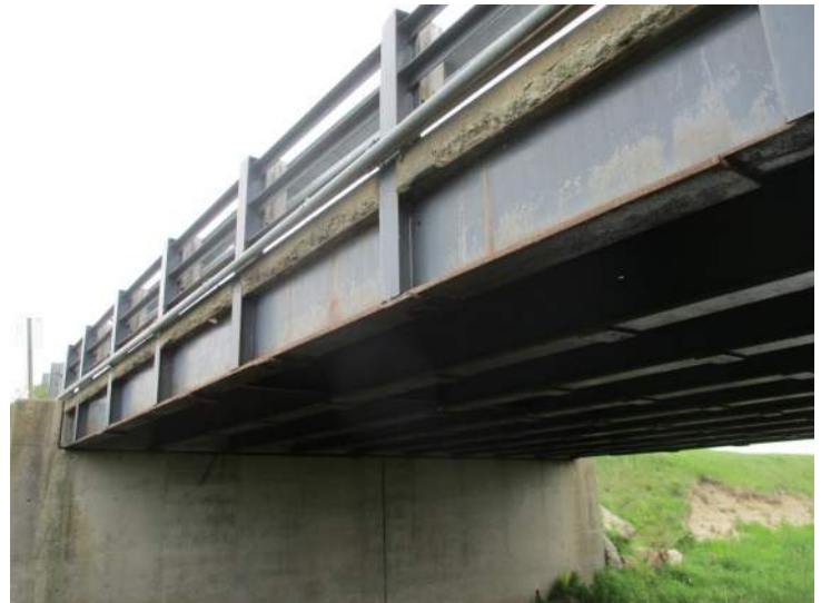
Document Name: 91.JPG Category: Elevation Span Number: Comments: South fascia, spalling
