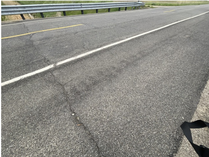
Document Name: IMG_9442.jpeg Category: Deck Span Number: Comments: Chip sealed HMA surface
